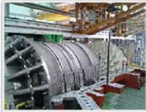
Blade Ring Dismantling, Lifting
