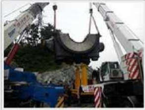
Seating the Exist LP Lower Casing
