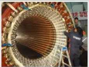
Dismantling of the Generator
